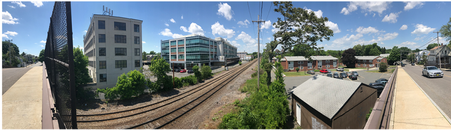
1 PANORAMIC VIEW FROM NORTH ST BRIDGE
