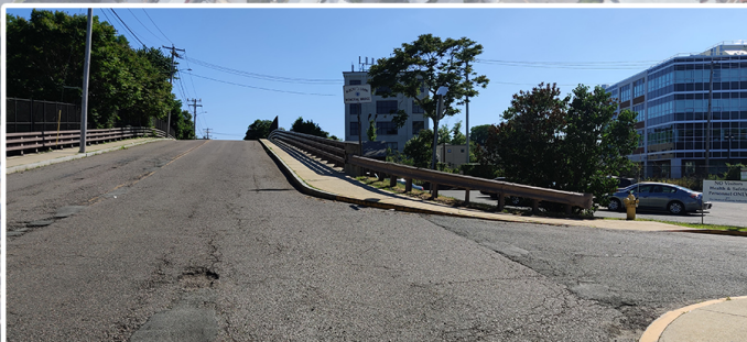
5 NORTH ST BRIDGE OVER MBTA TRACKS
