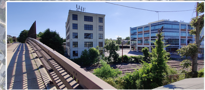
6 VIEW OF TRACKS FROM NORTH ST BRIDGE
