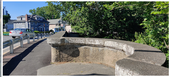
5 RIVER OVERLOOK ON PARKWAY
